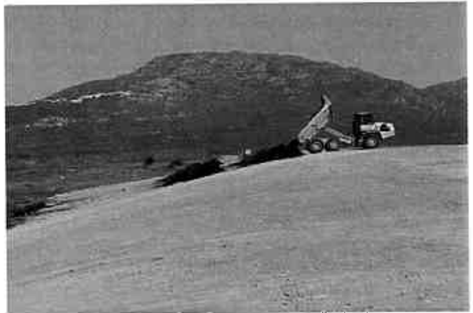
TOPSOIL BEING PLACED OVER CLAY CAPPING
